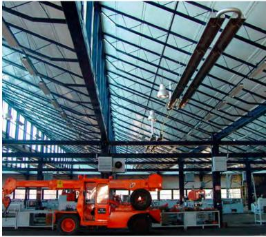
The double linear radiant tube needs reduced perforation of the building because it uses only one fan for two radiant tubes.
