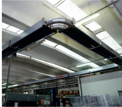
Radiant heaters with possibility to install the burner and gas line outside the building to avoid having to make holes in the roof for chimneys. Ordinary maintenance is carried out outside the building without having to interrupt the activity of the company.
