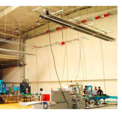
The radiant tubes directly radiate surfaces and people offering perfect thermal comfort even in buildings of great volume, and are also equipped with heat emitting tubes that allows them not to use paints that over time could detach from the pipe.
